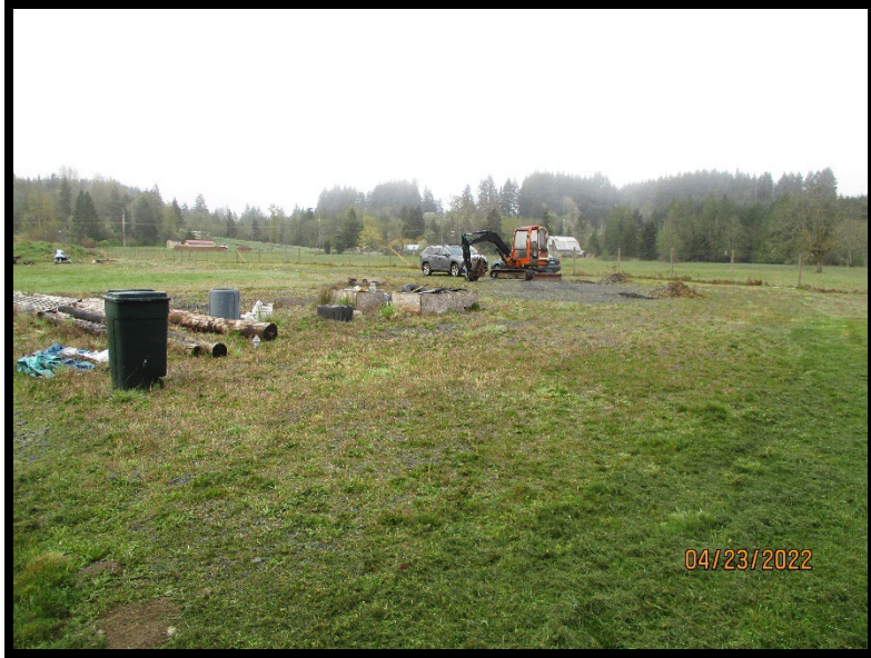
Photograph 2: Existing pad with excavated test holes. Looking southwest.
