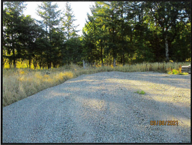
Photograph 1: Eastern extent of existing gravel pad.
